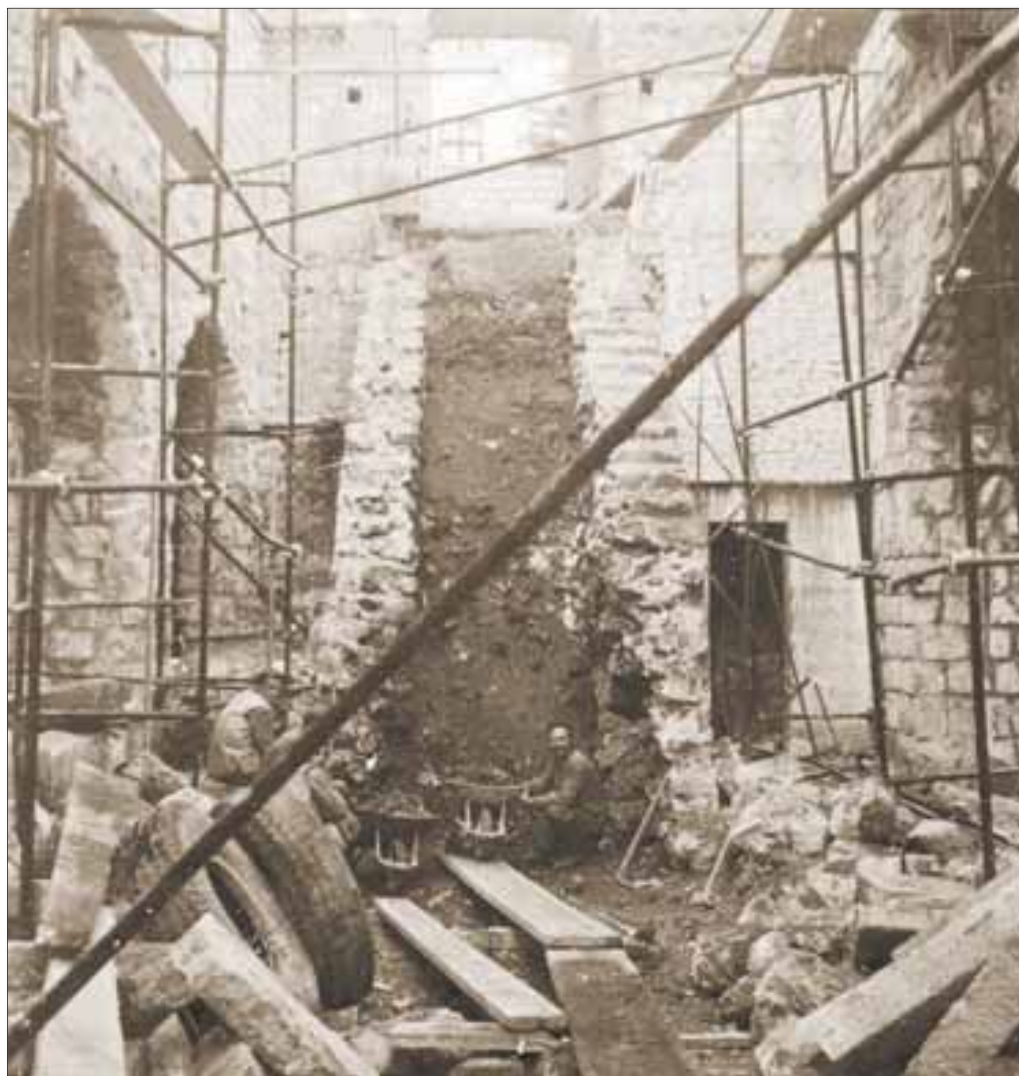
Fig. 19. Lazaretto during renovation, 1968
