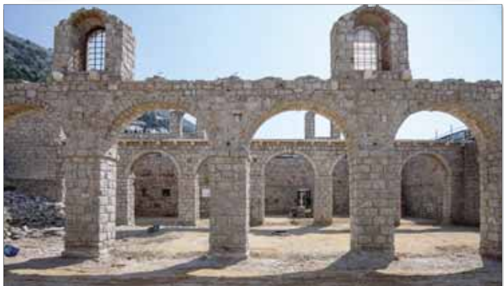
Lazaretto complex during restoration, 2018 (photographs: Institute for Restoration of Dubrovnik)
