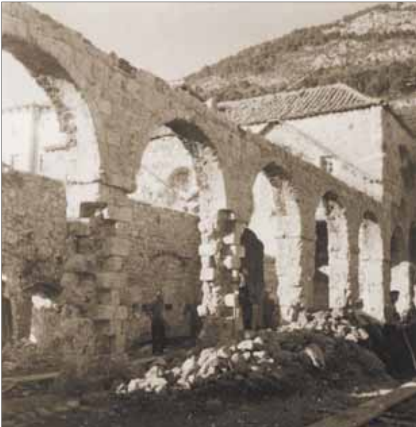
Fig. 18. Lazaretto during renovation, 1967-1969
