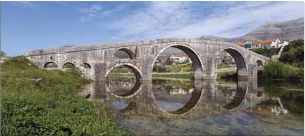
Fig. 5. Arslanagić Bridge, Trebinje, Bosnia and Herzegovina
