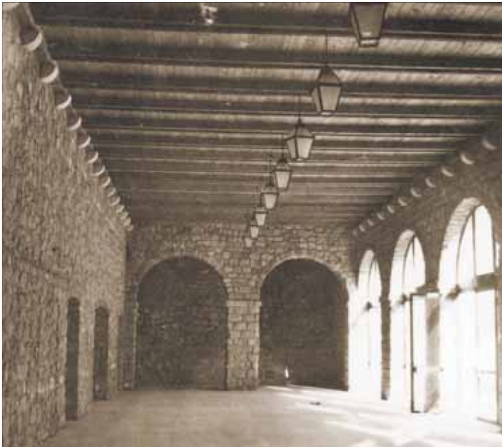
Fig. 20. Lazaretto after renovation, 1974
